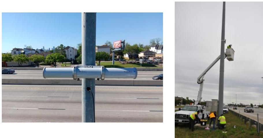
*Figure 8. Radar Detection Field Installation Examples*
