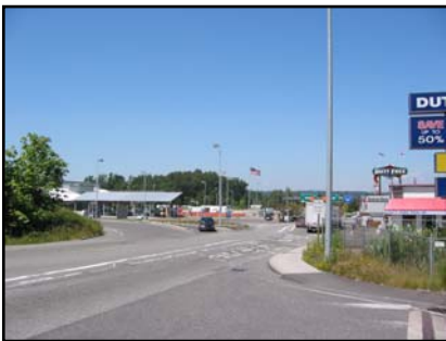
Looking northbound from the north end of the parking lot. U.S. passenger vehicle primary inspection booths at center left.
