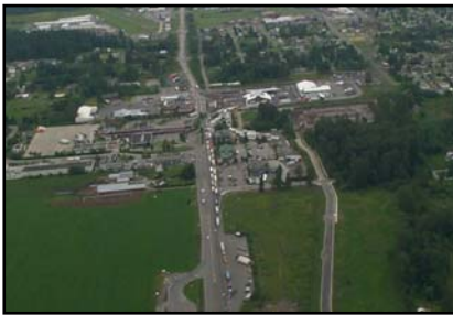
Looking southbound at Pacific Highway Border Crossing (prior to new gravel parking lot).
