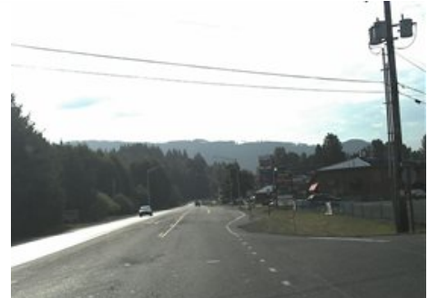
State Route 542 has paved shoulders and additional lanes for safety for turning vehicles near the Nooksack Tribal Head Start offices.
