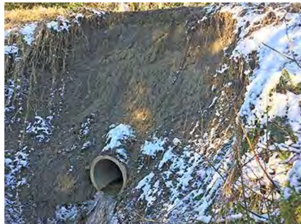
Above left: Photo shows scale of fish barrier at the outlet of the culvert. Above right: Photo shows prior damage when the downstream end of the culvert failed and temporary repairs were made to prevent loss of the roadway.
