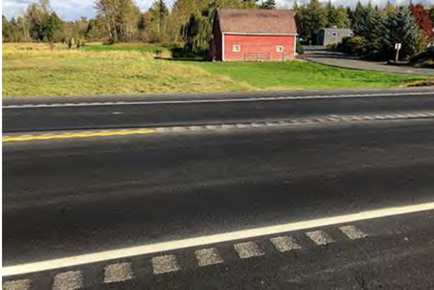
A pavement rehabilitation project completed in 2020 on Northwest Drive.
