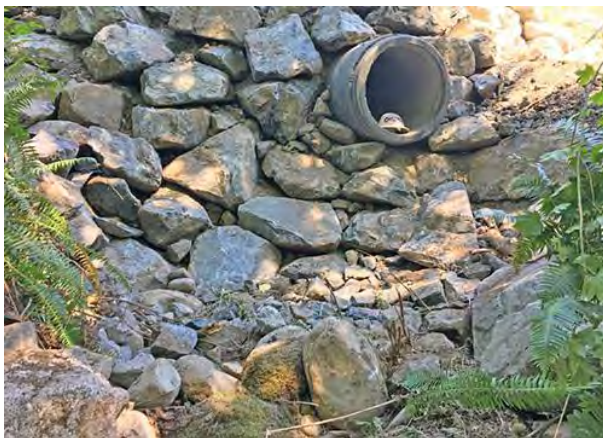
Above left: Photo shows scale of fish barrier at the outlet of the culvert. Above right: Photo shows prior damage when the downstream end of the culvert failed and temporary repairs were made to prevent loss of the roadway.
