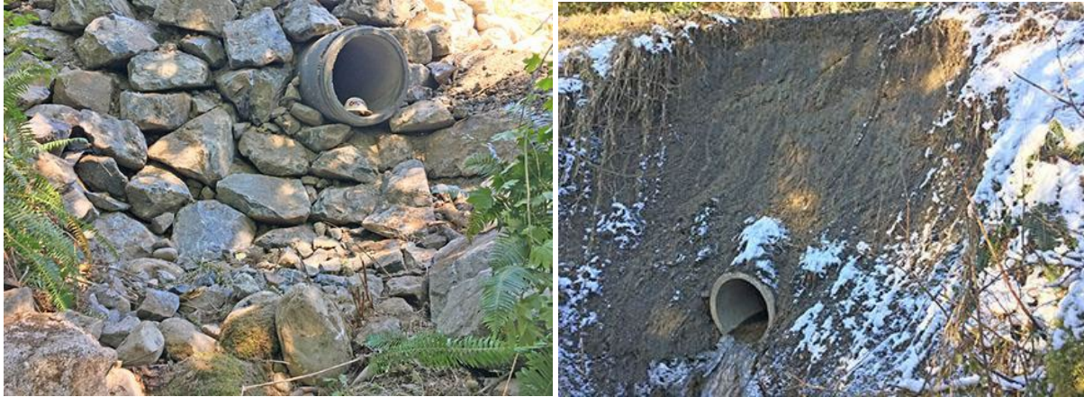
Above left: Photo shows scale of fish barrier at the outlet of the culvert. Above right: Photo shows prior damage when the downstream end of the culvert failed and temporary repairs were made to prevent loss of the roadway.
