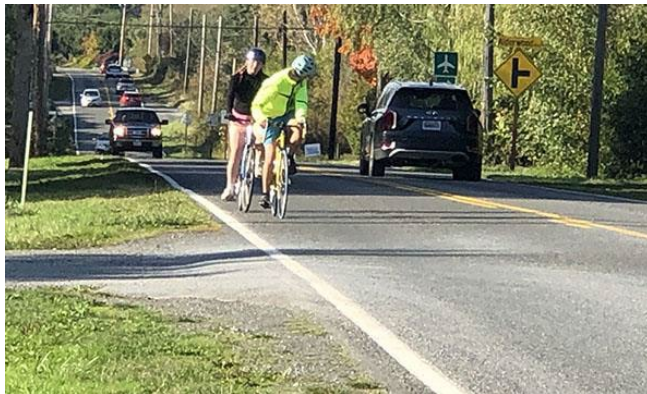
The lack of bike lanes and sidewalks – as well as inadequate or non-existent shoulders – makes bicycling and walking hazardous in many locations along Marine Drive.
