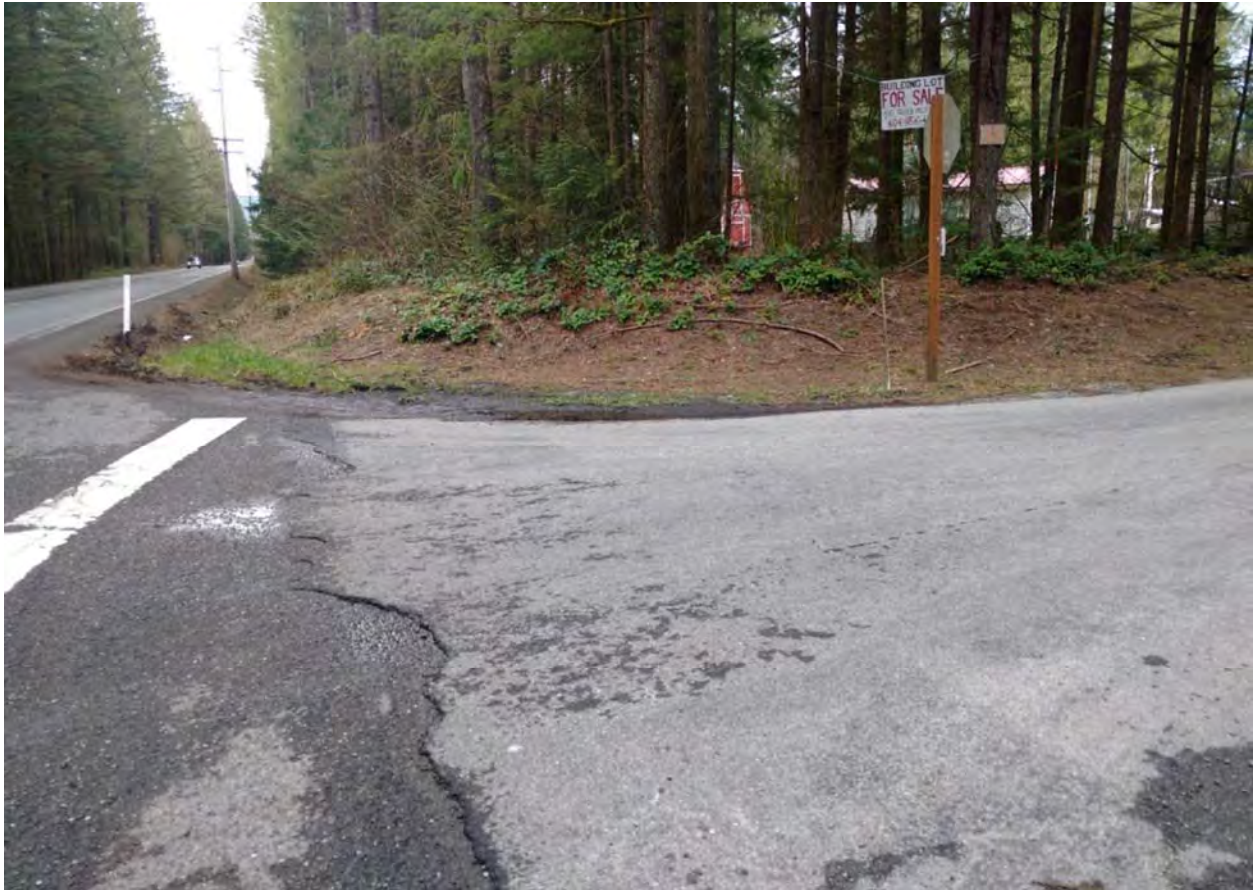
72X Kendall – Peaceful Valley Dr. at Kendall Rd - proposed bus stop shelter.
