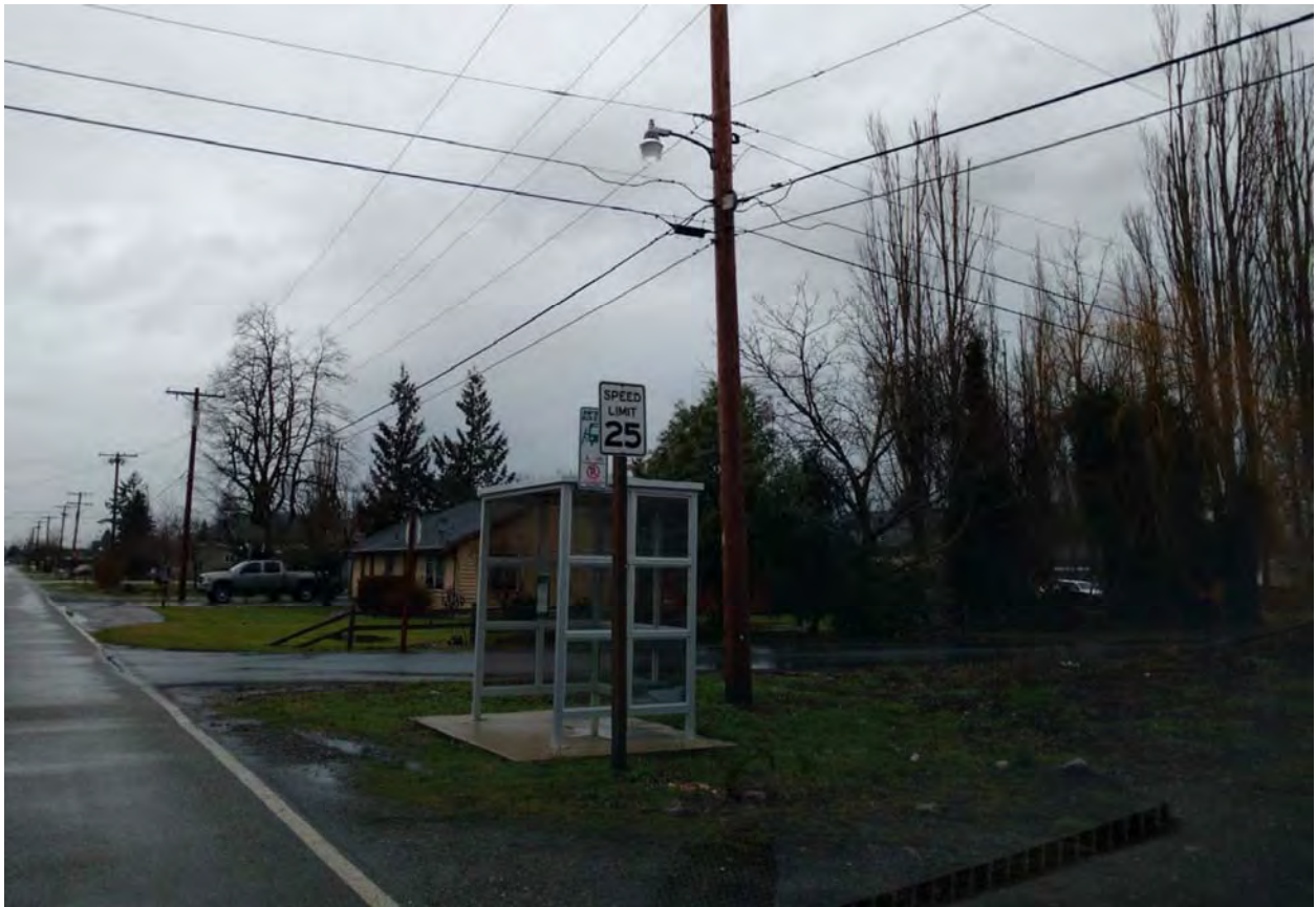
71X Sumas – Sumas at Morton Inbound - proposed concrete pavement from shelter to roadside.
