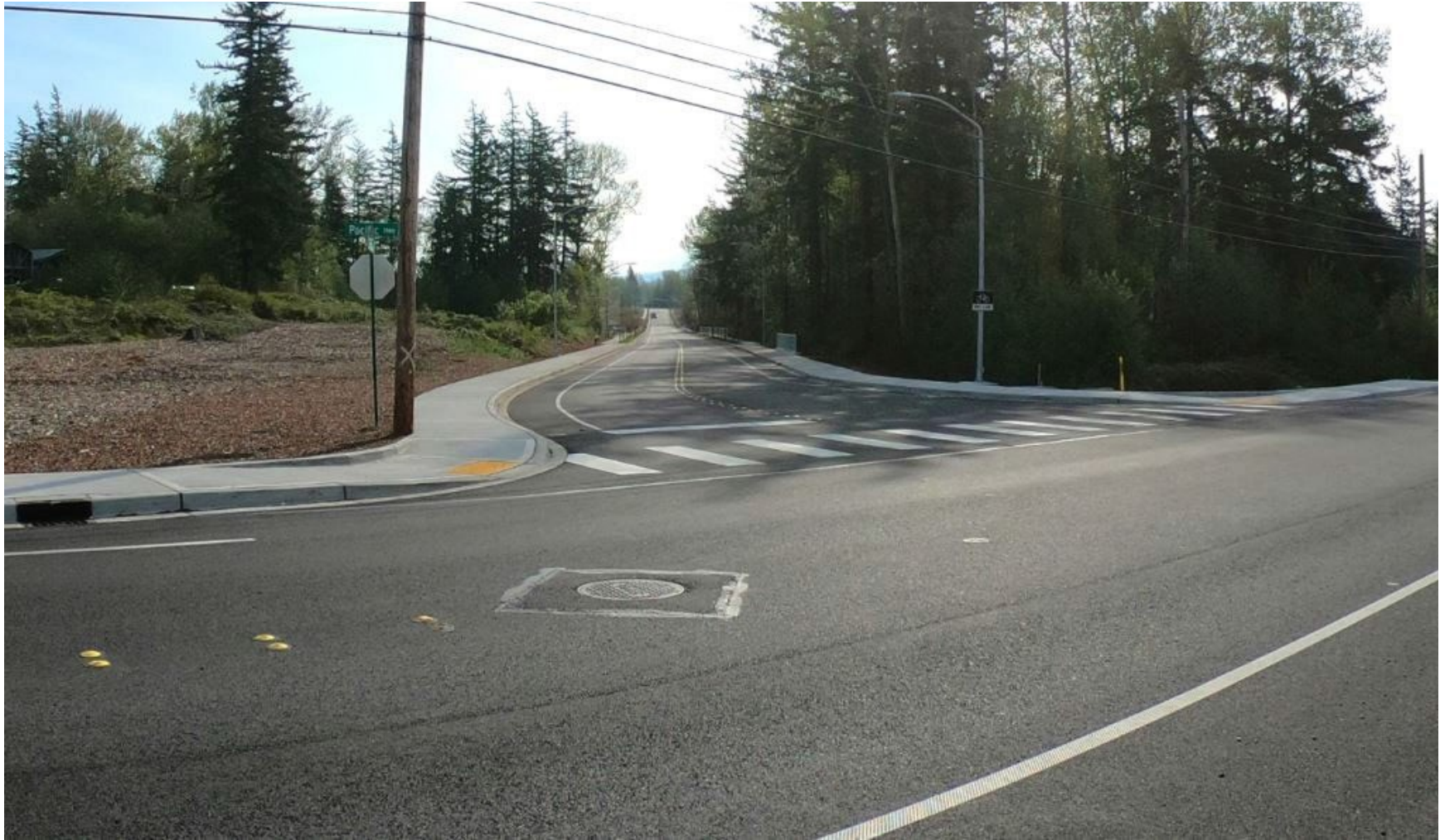
Mahogany Ave connects Pacific Highway to Arctic Ave and Northwest Dr in the growing northern section of Bellingham.
