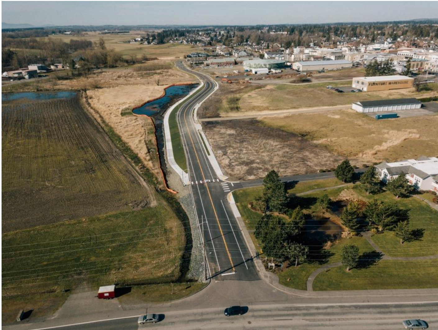
Completed in 2019, Riverview Road construction in Lynden completed a multimodal connection between 6th St in downtown to Hannegan Road east.
