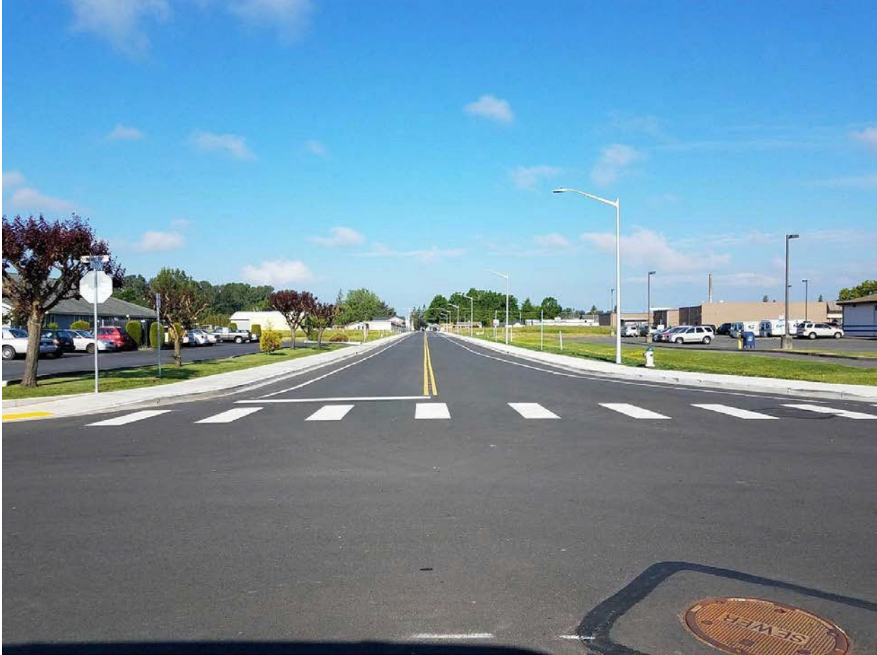
Opened in 2019, Everson’s Lincoln St was reconstructed from Everson Rd to Washington St and extended the roadway construction from Washington St to Blair Rd.
