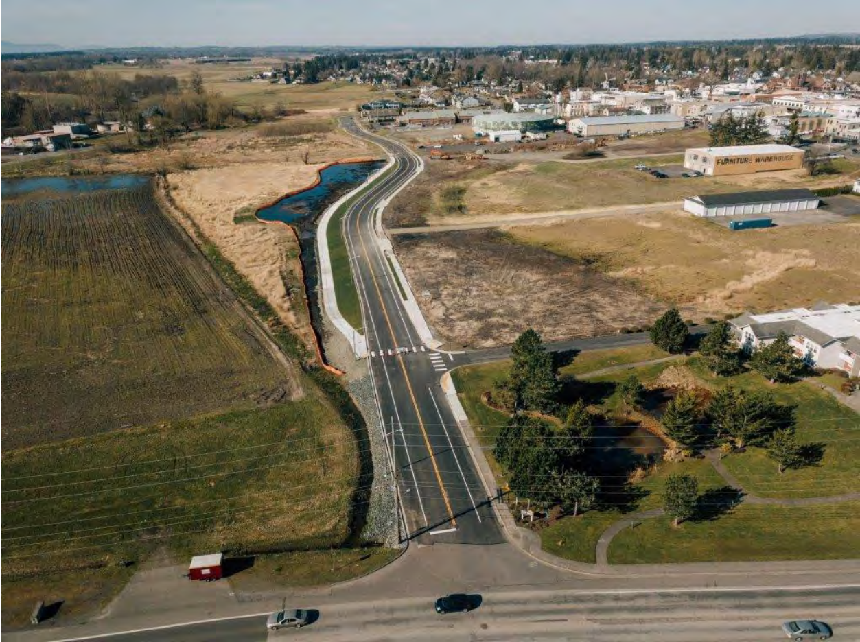
City of Lynden recently finished the new roadway construction of Riverview Rd that connects the S 6th St to Hannegan Rd.
