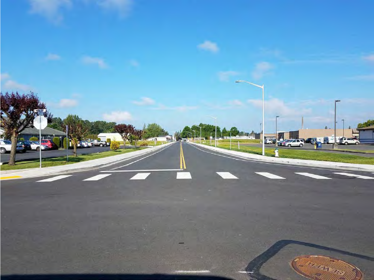
Opened in 2019, Everson’s Lincoln St was reconstructed from Everson Rd to Washington St and extended the roadway construction from Washington St to Blair Rd.
