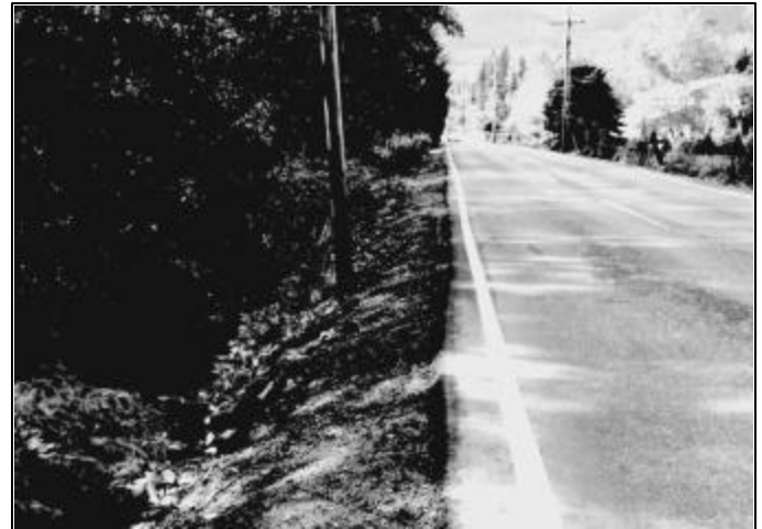
Figure 1 Narrow shoulders along Mt. Baker Highway
